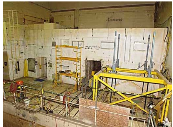
Fig. 2. Hot Cell 1 and 2 prior to Remediation Efforts.
