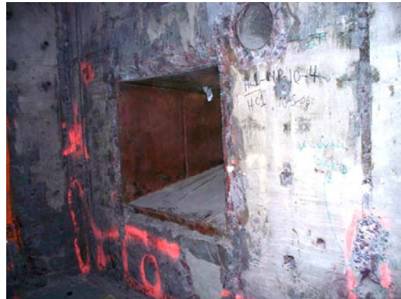
Fig. 6. Example of “Lunar Landscape” like surface resulting from initial remediation approach.
