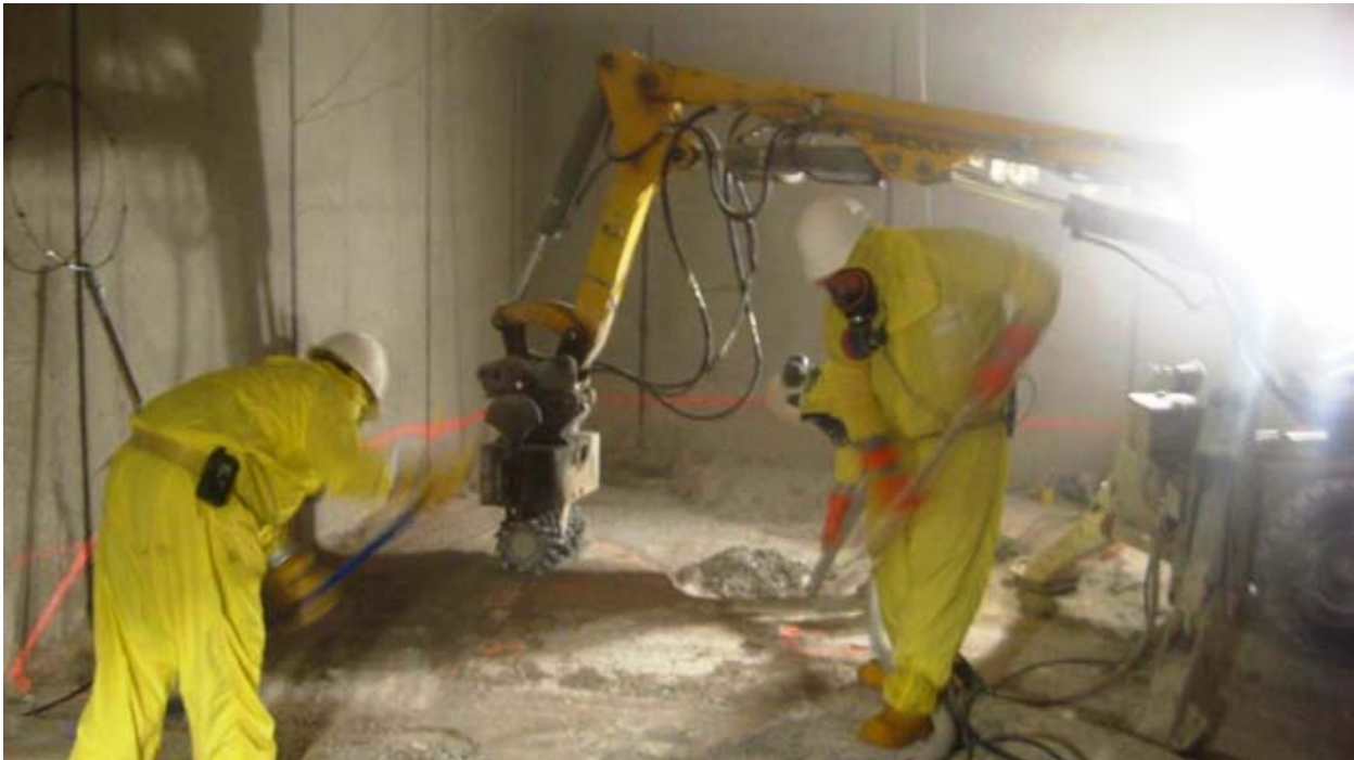
Fig. 11. Actual spot remediation efforts within the hot pipe tunnel.
