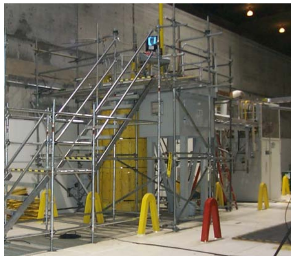
Fig. 2. A system for treating the NLOP sludge was set up in T Plant.
