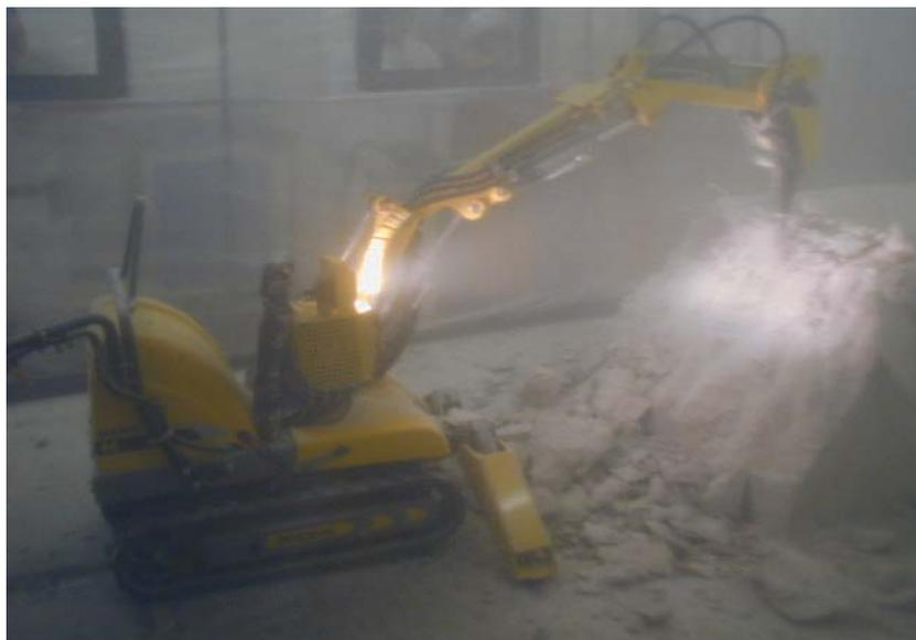
**Brokk 40 breaking out concrete plinth**
