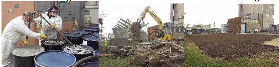
**4. Grouting cut pipes into 200L drums    5. Demolition of ABR structure    6. Landscaped site.**
