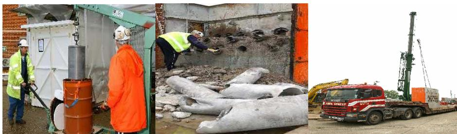
**4. Lead casket housing ILW segment of BP    5. Monitoring surfaces of storage pockets    6. Outer steel casing ready for transport off site.**
