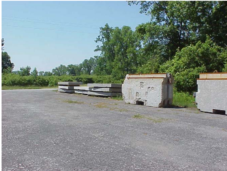
Fig. 17. Hot cell roof slabs and inter-cell transfer doors after release from the site
