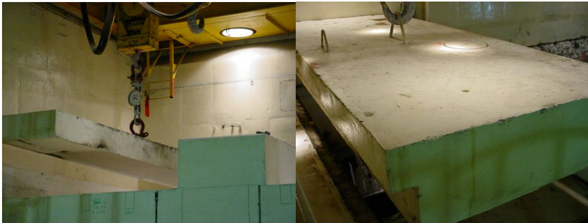
Figs. 7, 8. Removal of hot cell roof slab using installed overhead crane.
