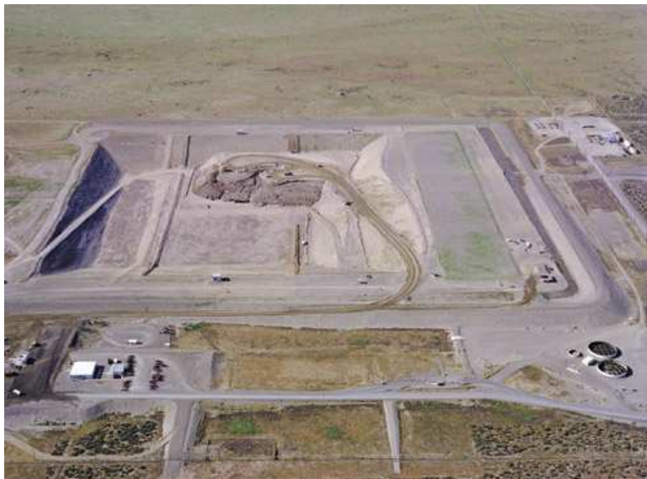
Fig. 1. An aerial view of Hanford's Environmental Restoration Disposal Facility.
