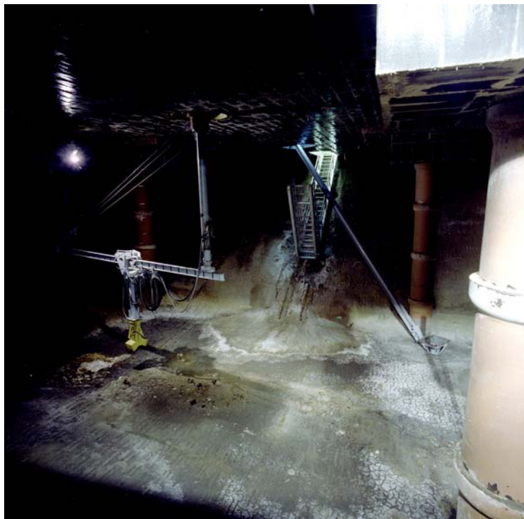
Figure 2. Historical View, Z-9 Crib Mining Equipment
