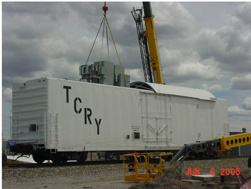
Fig. 2. Load out of Large Equipment on the Beer Can Express
