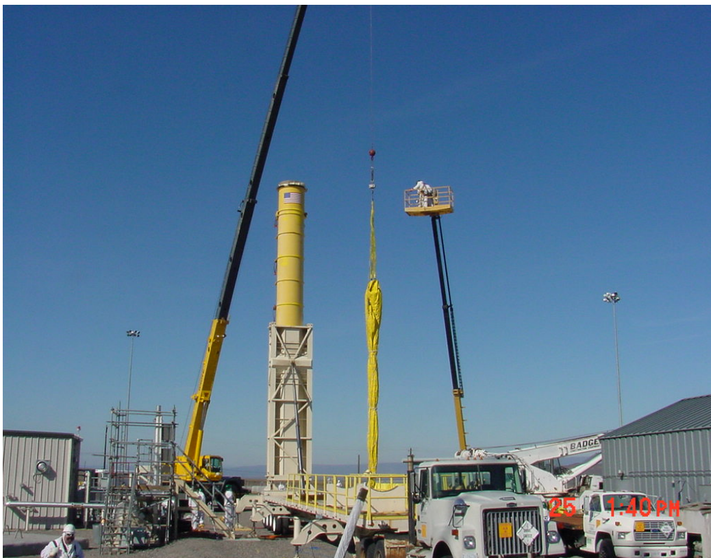
Fig. 1. Testing of the Long Length Equipment Retrieval, Packaging, and Transport System
