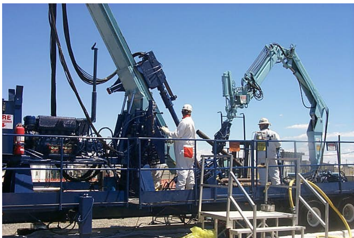
Fig. 1. Diesel hammer drill rig in SX Tank Farm
