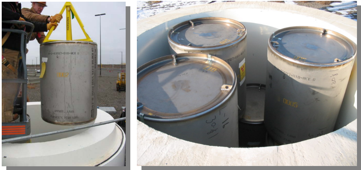
Fig. 5. Packaged overpack placement into the RadVaults.
