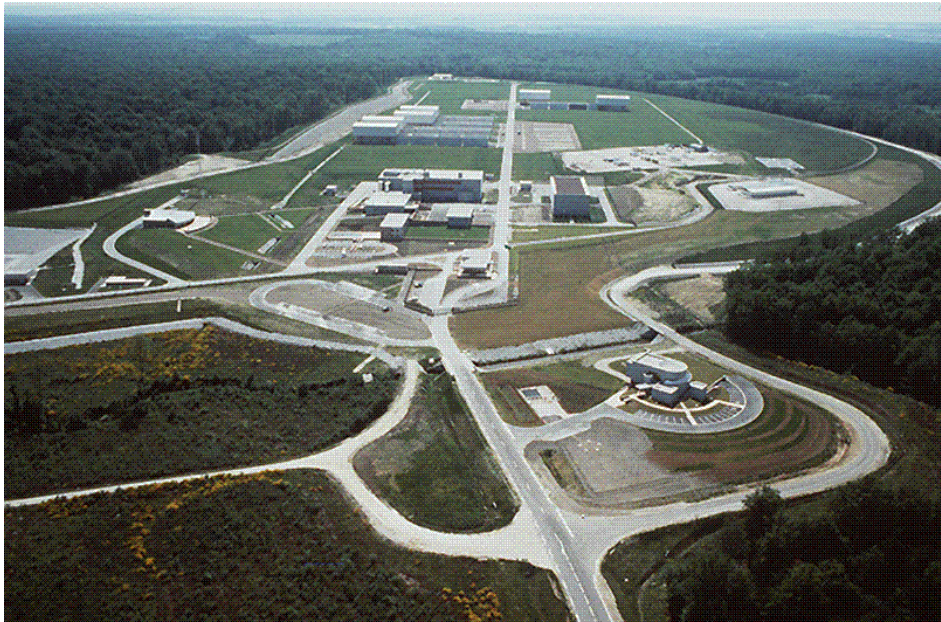
Fig.2. Centre de l’Aube disposal facility for LILW
