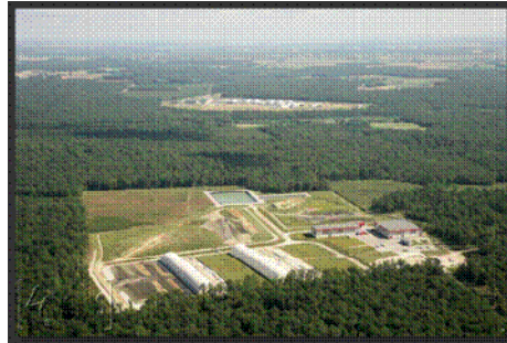
Fig.3. Aerial view of the Centre de Stockage Tres Faible Activite in Morvilliers
