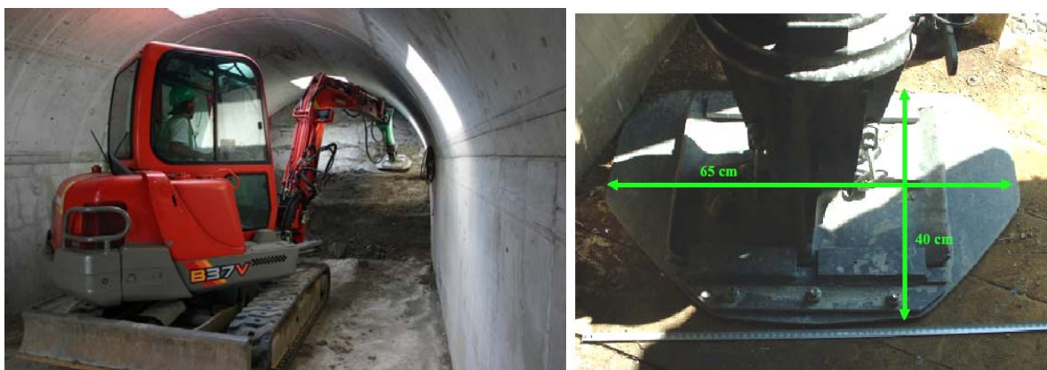
Figure 2. Hydraulic percussion rammer mounted on a power shovel.
