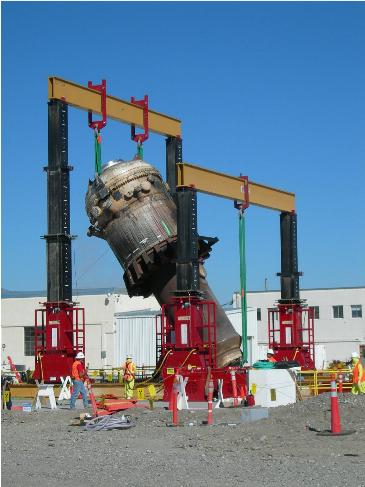
Fig. 3. The 112-ton Engineering Test Reactor vessel was removed and subsequently disposed at the ICDF.
