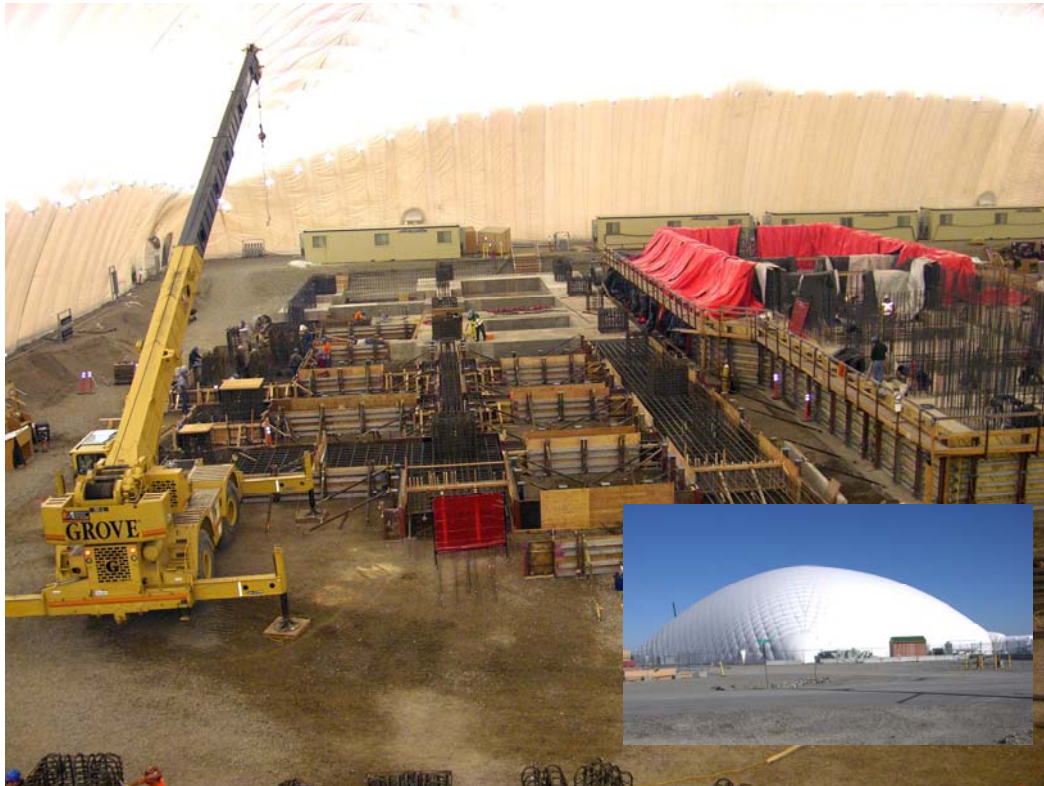
Fig. 4. Weather enclosure allows IWTU construction to continue during winter months
