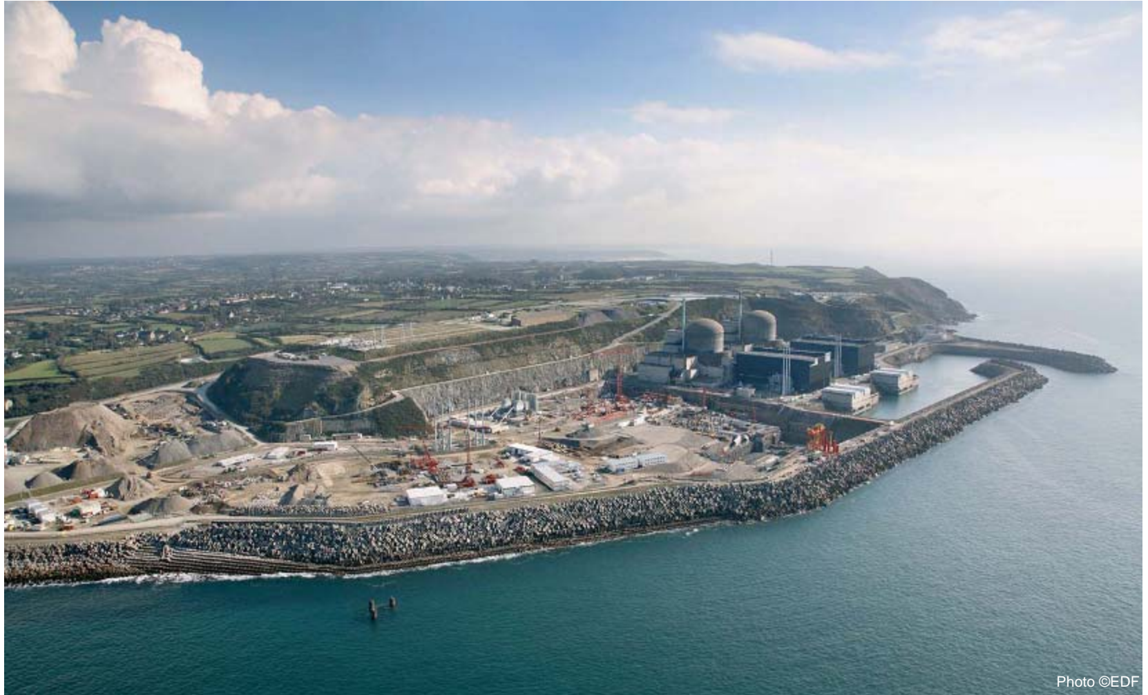
Flamanville 3 Project: January 2008
