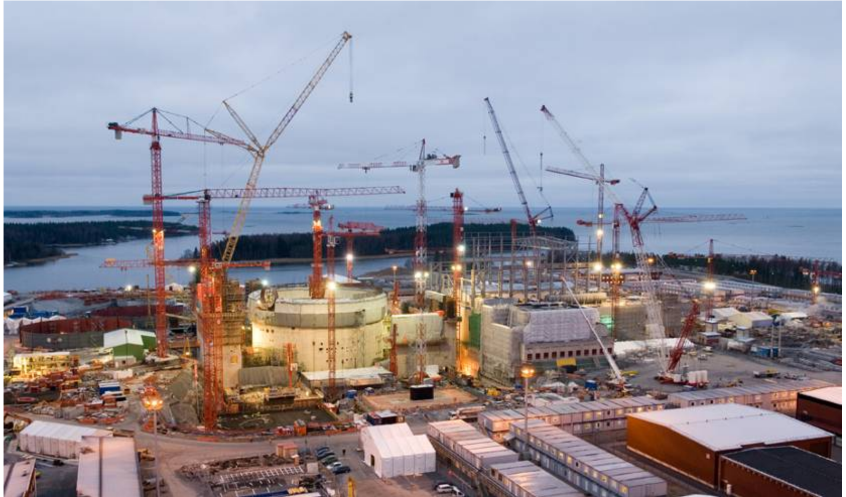
Olkiluoto 3 Project: January 2008
