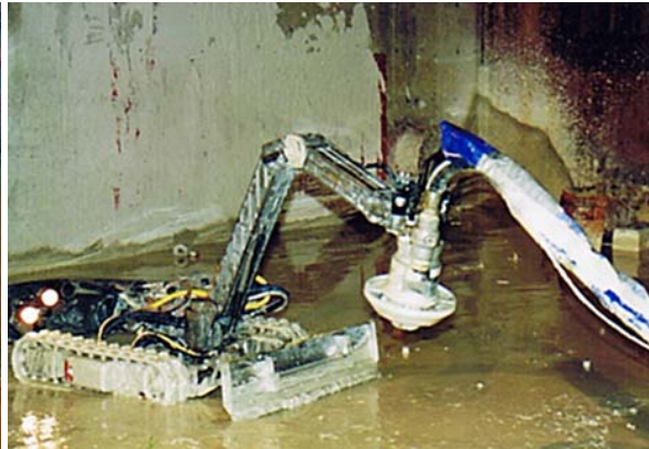
Retrieval of tank waste
