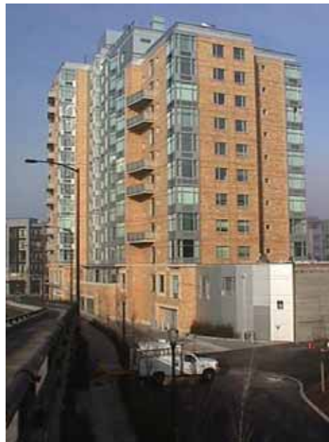
Fig. 2. Station place residential tower on Lot 1, following construction.
