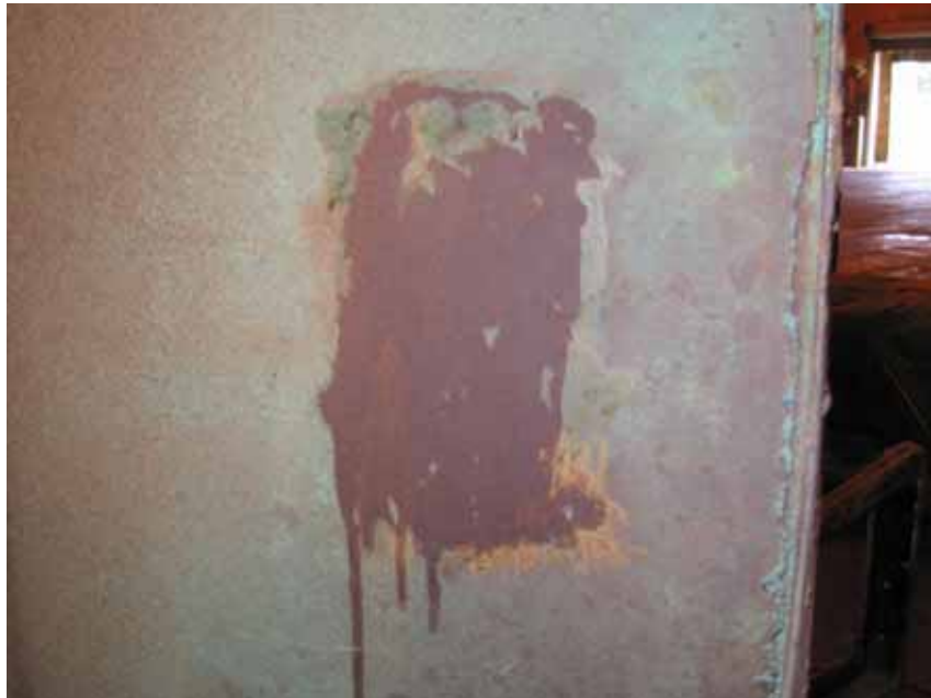
Figure 1 - Oxidized steel after decontamination
