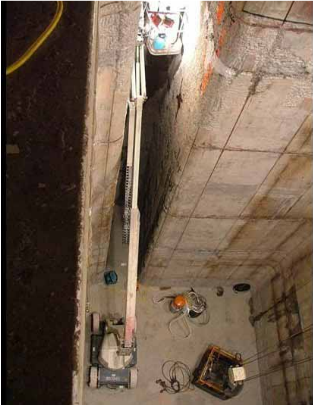
Figure 2. Closure Services successfully removed the stainless steel liner and surface released the fuel basin extending 50 feet below surface grade and avoiding costly excavation of the structure.
