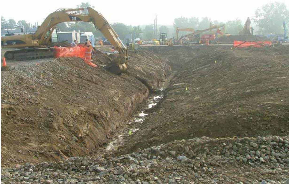
Figure 3, Closure Services minimized the waste volume of soil surrounding the underground-contaminated lines that were removed by using a CS procedure approved by the U.S. NRC.
