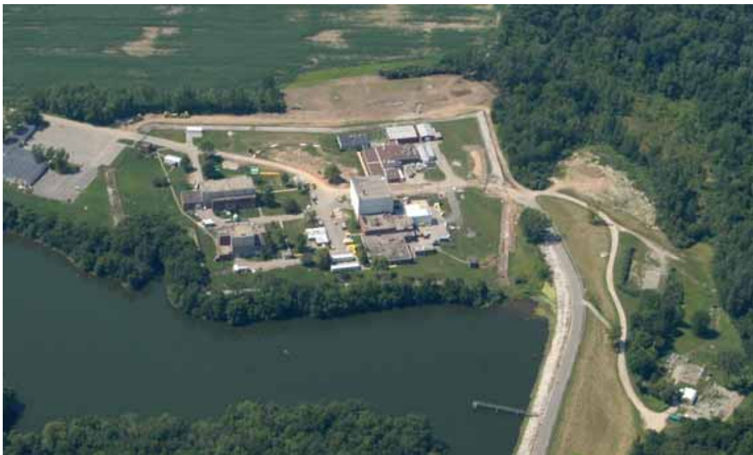
Figure – 1. The Columbus Closure Project site buildings previously contained a retired 2 mega-watt research reactor, a plutonium test facility and radioactive material analysis laboratory, three large hot cells, and contaminated 50 ft fuel pool basin.
