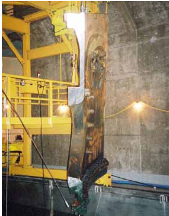
Fig. 3. Core support shield segment.
