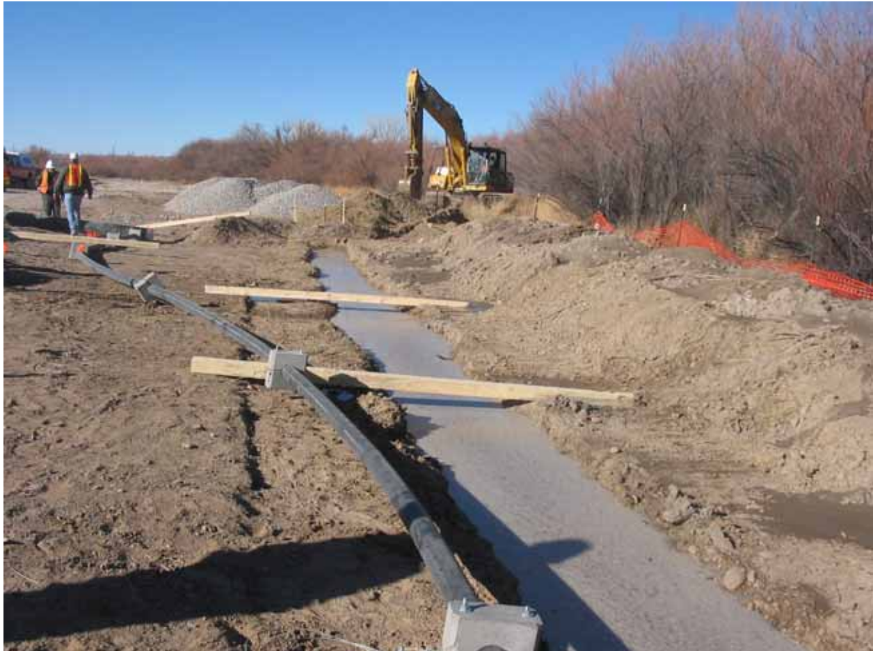
Fig. 4. Guar-gum-based construction of collection drain.
