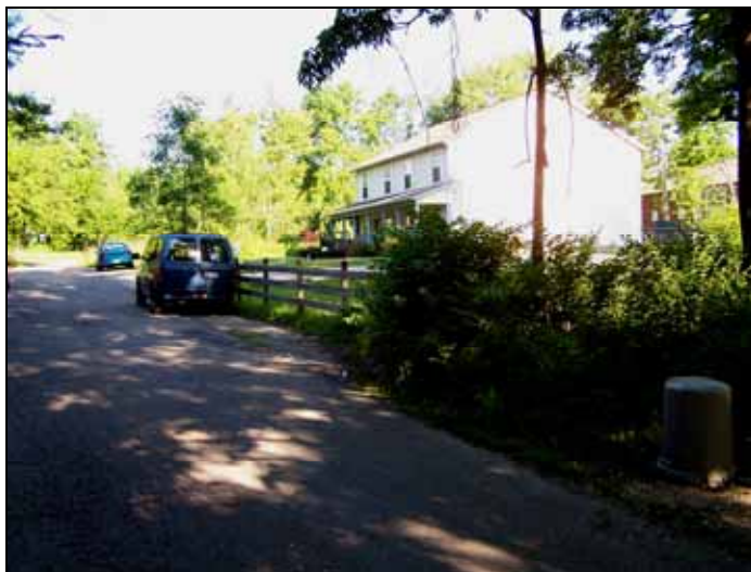
Fig. 5. The Alba Craft Laboratory at the Oxford, Ohio, Site, was razed and a duplex was built on a portion of the property.
