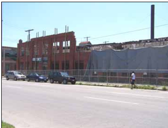
Fig. 4. The Columbus East, Ohio, Site (B&T Metals) may be redeveloped for any land use because the site was released without restrictions.
