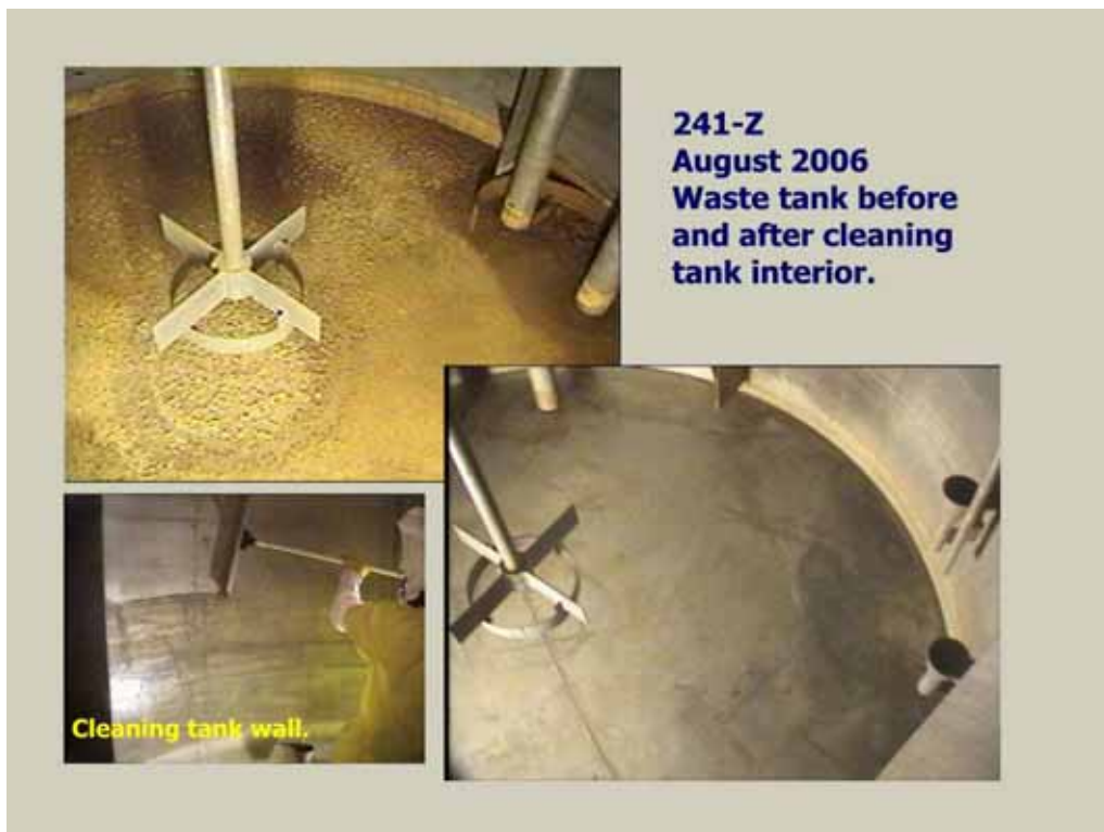
Figure 4 - RCRA closure activities: cleaning tank interior
