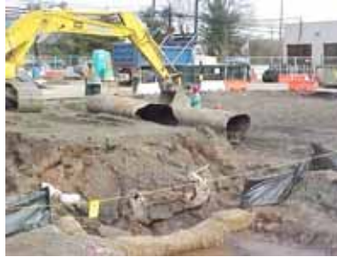
Fig. 2. Removal of historic ECMP sections at the 160/174 Essex Street property.
