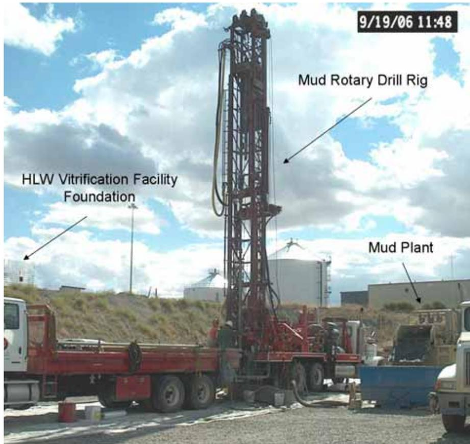
Fig. 5. Mud rotary drilling of borehole C4993.
