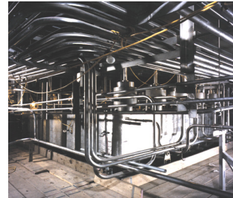
Mixer settler stirrer shafts under PSC Roof
