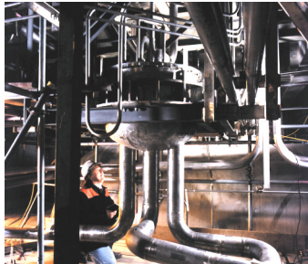
In-Cell Liquid Distributor
