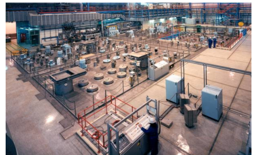
Typical Type 3 PSC roof with stools and gamma gates in position
