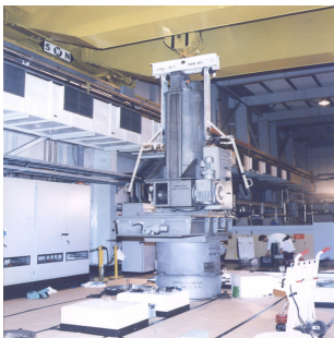
Flask, gamma gate & stool in place on Type 3 PSC roof
