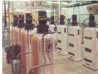
Mixer settler stirrer motors on PSC Roof
