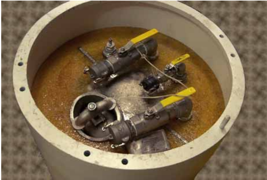
Fig. 4. DT-355 Encapsulation Container before closure cap is poured.
