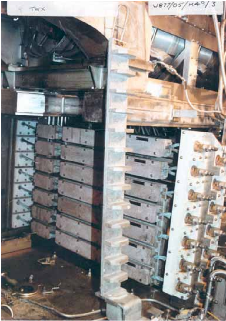
Fig. 1. View of the through wall crossings inside cell
