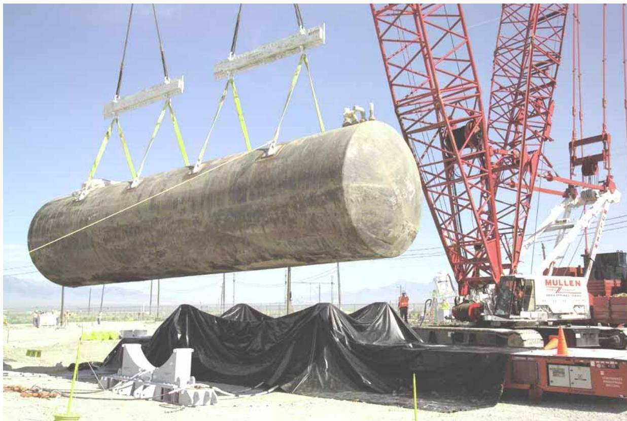
**Fig. 1. Removal of a PM-2A tank from its original location at TAN.**
