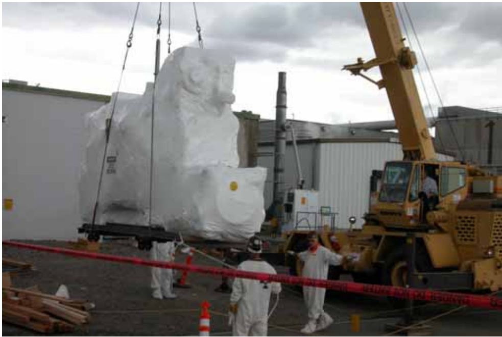
Figure 3. After the internal equipment was removed from the incinerator glovebox, the glovebox was packaged and removed from the facility to be size reduced at the Hanford size-reduction facility at T-Plant.
