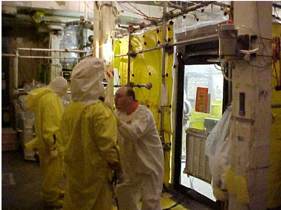
Figure 4 – Prior to entering the scrubber cell access tent, a final check of PPE is conducted and the fresh air breathing hose is attached. Monitoring of the airborne environment, conducting aggressive ash fixing processes and performing extensive checks on protective equipment resulted in 104 safe entries into the highly contaminated scrubber cell room.
