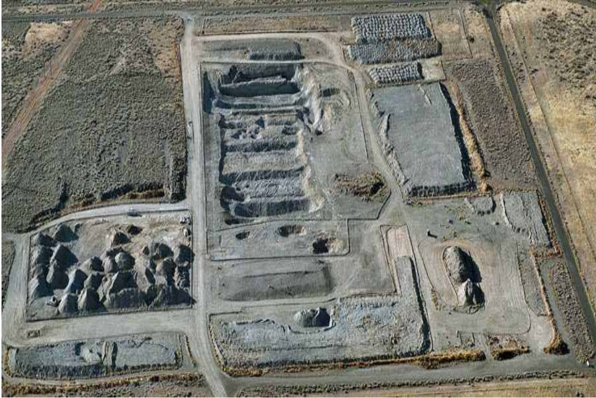
Fig. 3. 118-B-1 Burial Ground (100-B/C Area) under remediation, looking south.
