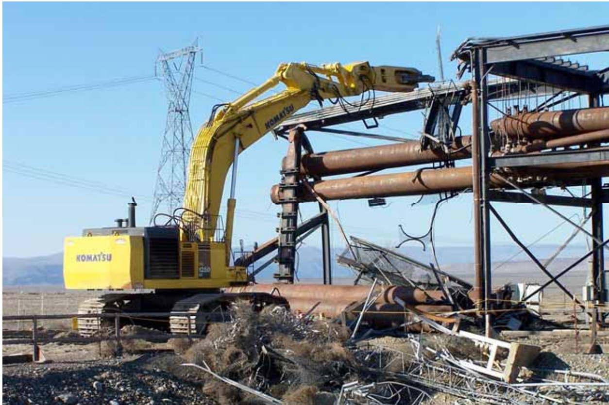
Fig. 2. Demolition of the 1802N pipe trestle at Hanford's N Reactor facility
