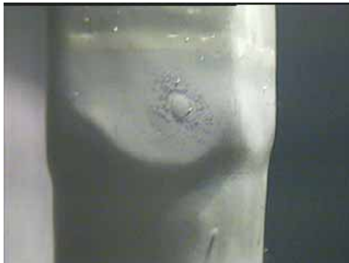
Fig. 2. Visual inspection on determination of parameters 6, 10 and 11.
