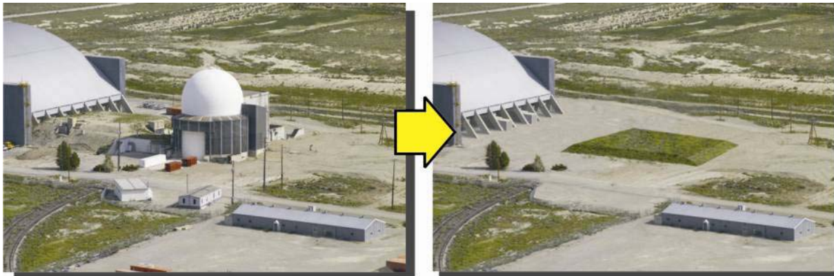
Fig. 4. D&D crews on the Idaho Cleanup Project used unique D&D techniques to deliver the LOFT demolition safely while preserving a historically significant part of the reactor development era.
