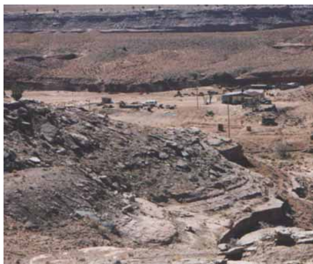
Figure 2. Navajo house adjacent to a uranium mine in northern New Mexico. Radioactive waste rock from uranium mine (now reclaimed) in left foreground of picture was used to build foundation for house shown in upper right. The house was subsequently reconstructed by the Navajo Nation to remove contaminated building materials.
