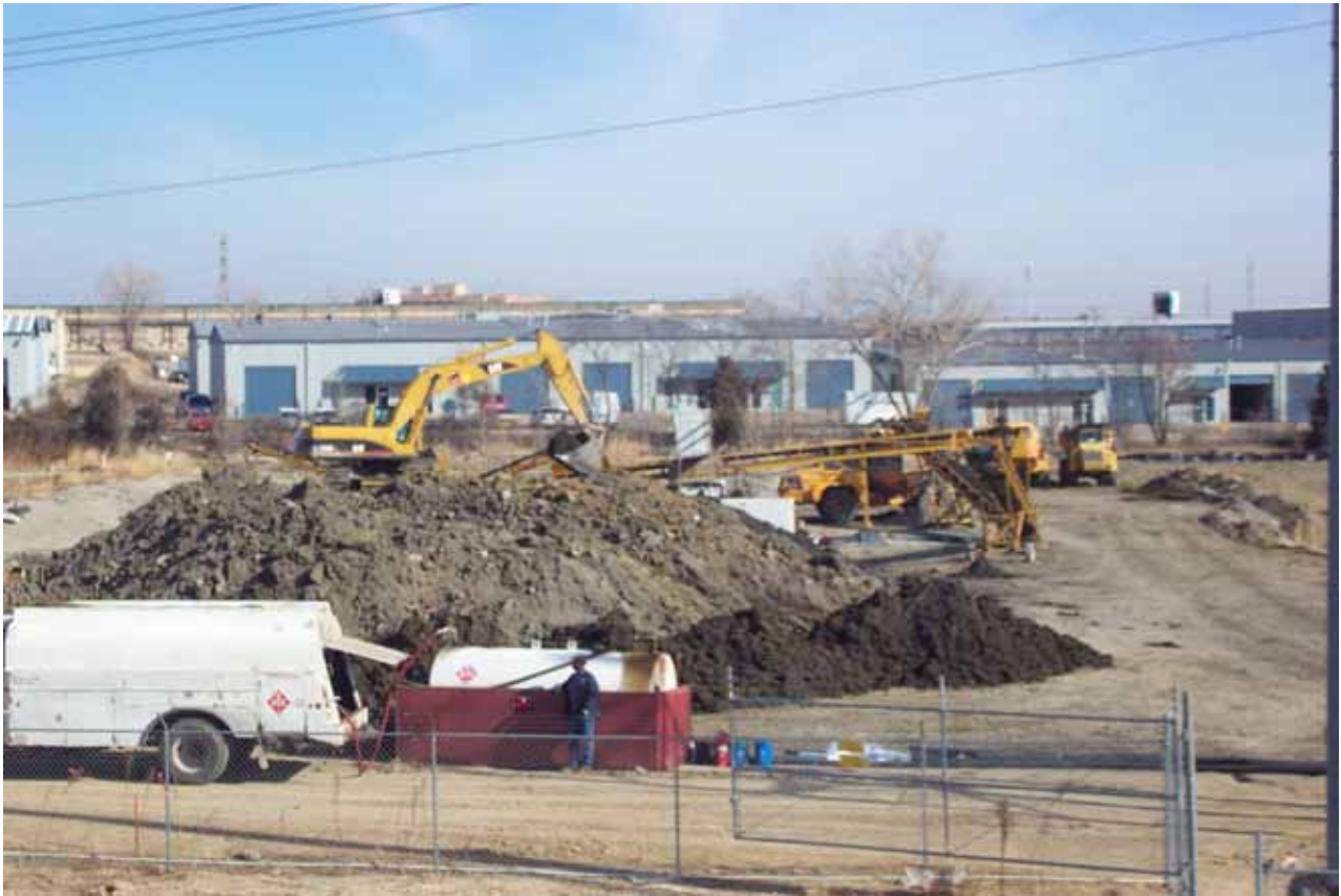
Fig. 2. Segregation system view B
