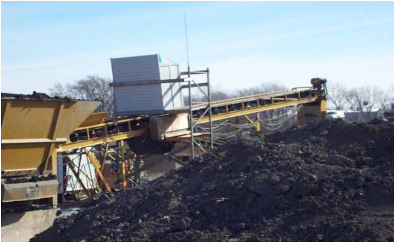
Fig. 4. Segregation system detector dog house
