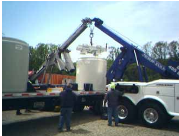
Figure 4. Transfer of casks to new trailer using 2 tow trucks.
