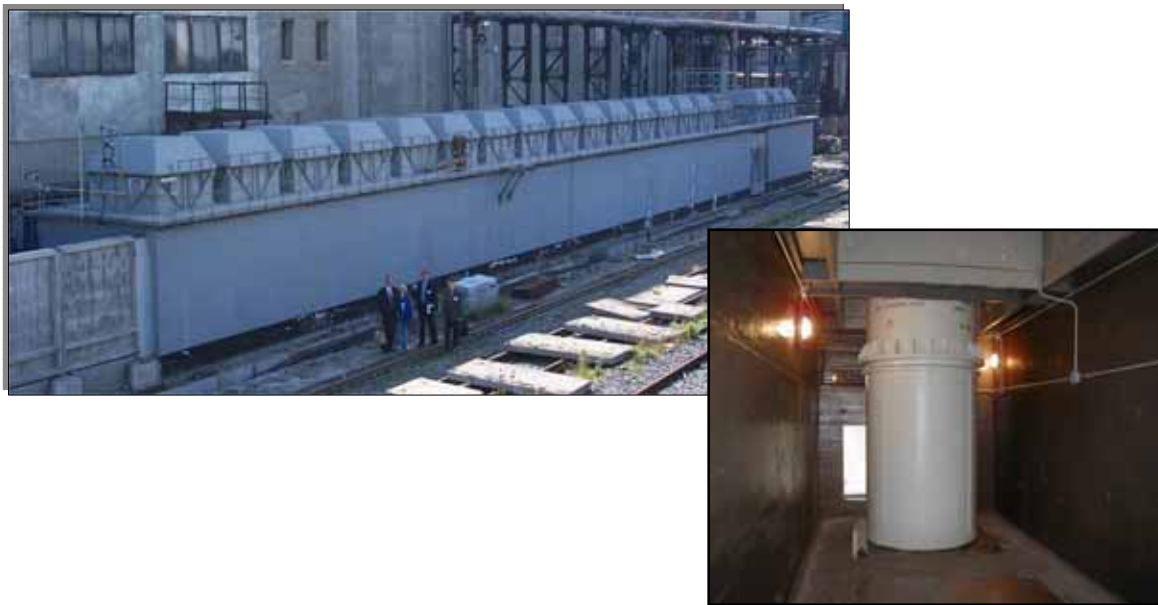
Fig. 3. Completed Transshipment/Interim Storage Facility with the TUK-108 Prototype Cask in one of the 19 storage positions
