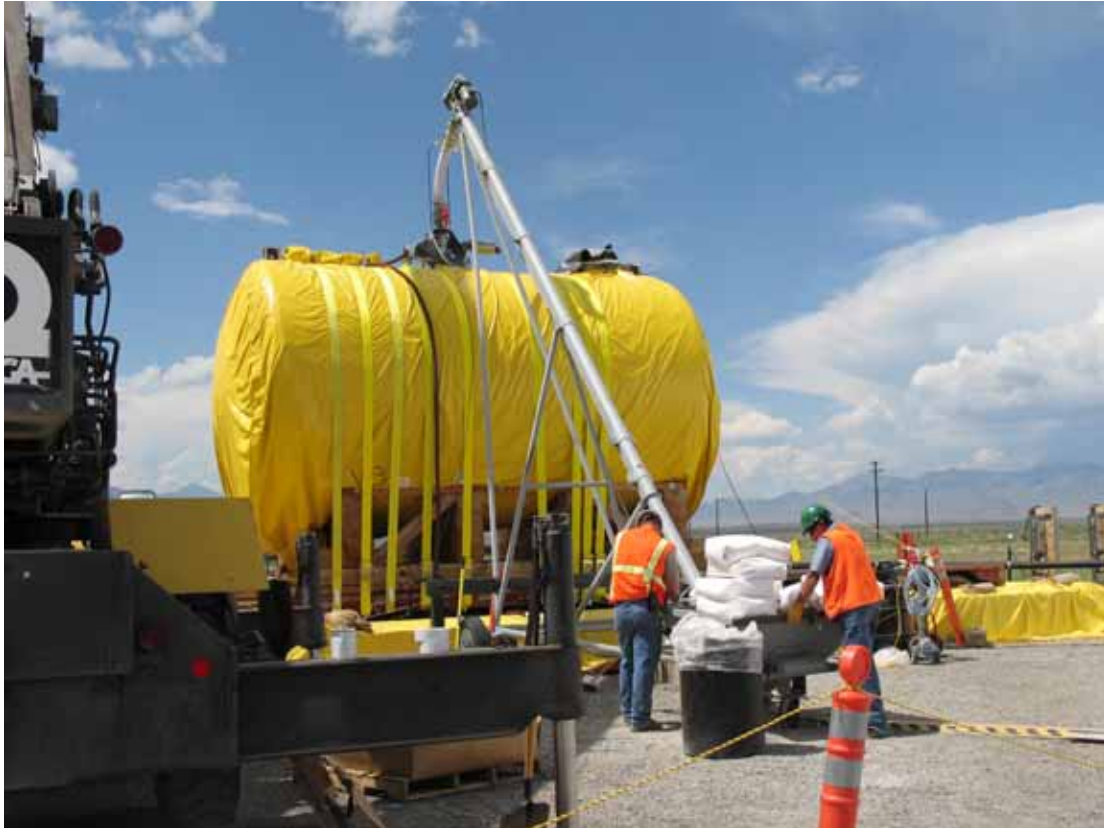
Fig. 2. Solidification system used for the consolidated V-Tank waste.
