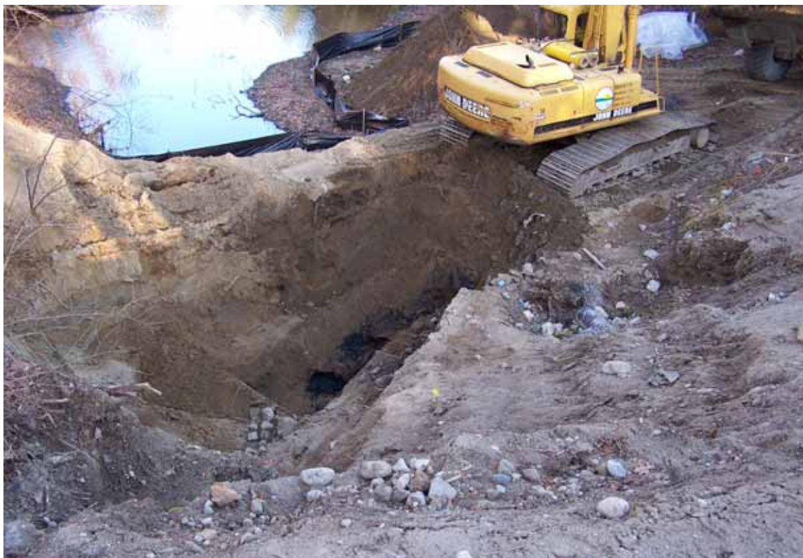
Figure 2. Former Drum burial area excavation
