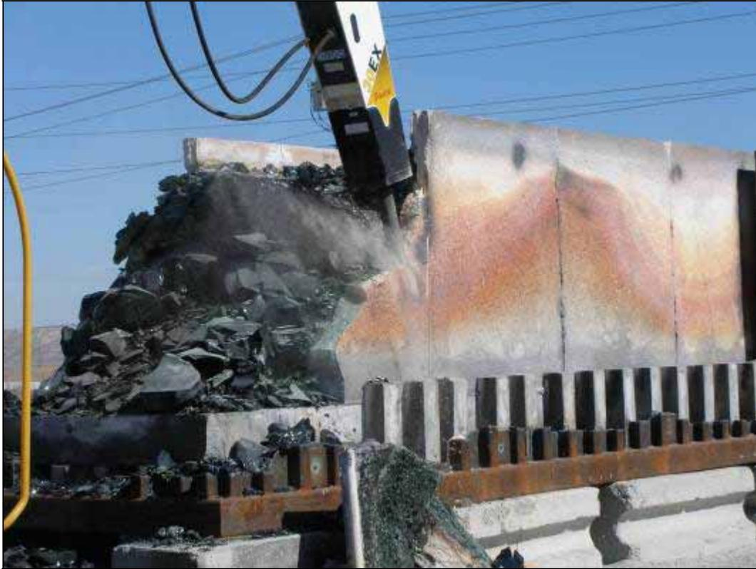
Fig. 4. Post-melt ICV™ container examination and dismantling.
