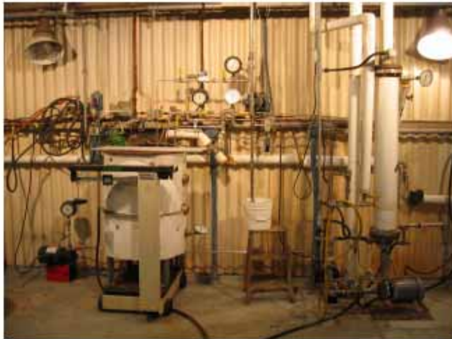
Fig. 8. Swenson DTE equipment – lower level.
