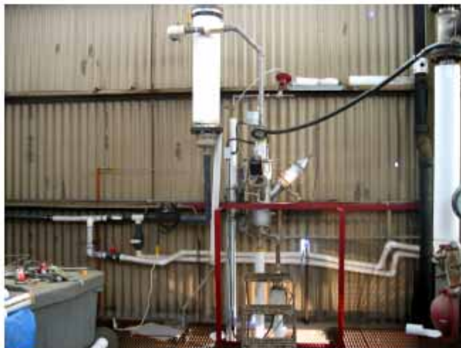
Fig. 9. Swenson DTE crystallizer and condenser – upper level.
