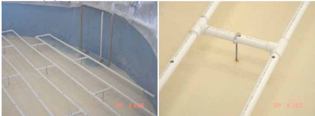
Figure 3: Tank condition after heel retrieval. Outline of 3/8” cooling coil support plates were clearly visible.
