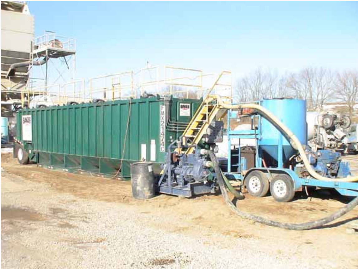
Figure 2: Bentonite mixing and hydration tanks at the offsite concrete batch plant
