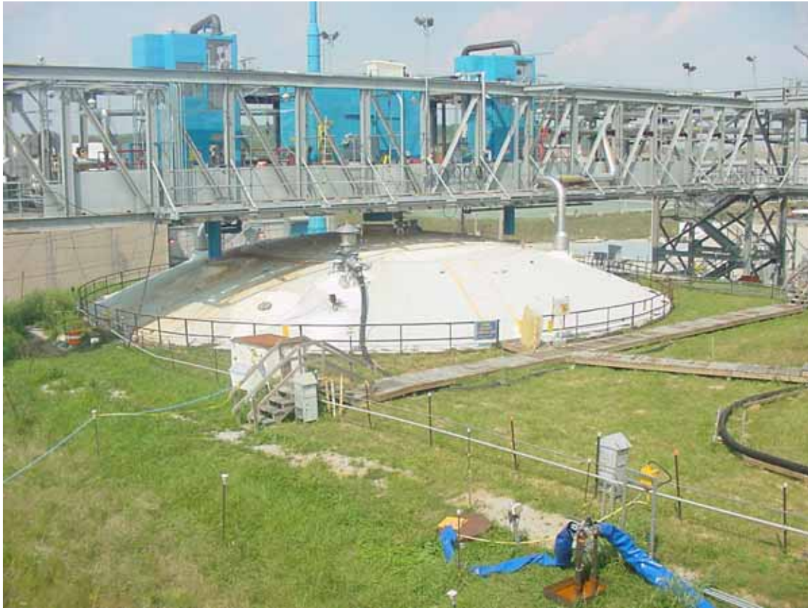
Figure 1: Exposed dome of silo 1 with bridge mounted blue containment modules
