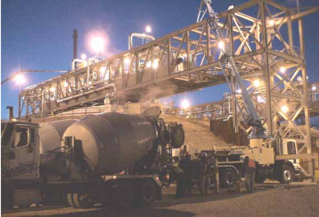
Figure 3: Silo 2 pumping begins at dawn on north side
