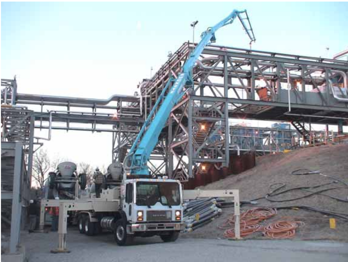
Figure 4: Silo 2 pumping operations at southeast side
