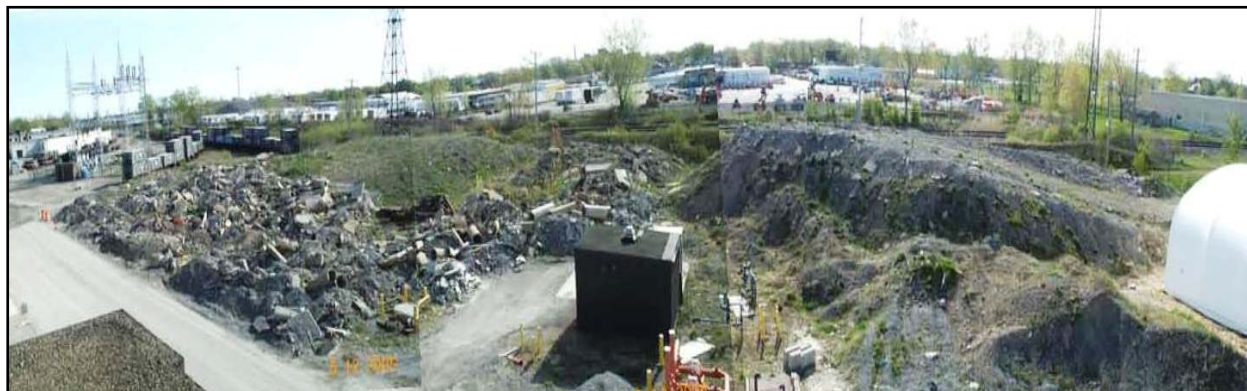
Figure 1 – Configuration of Spoils Pile – May 2005.
