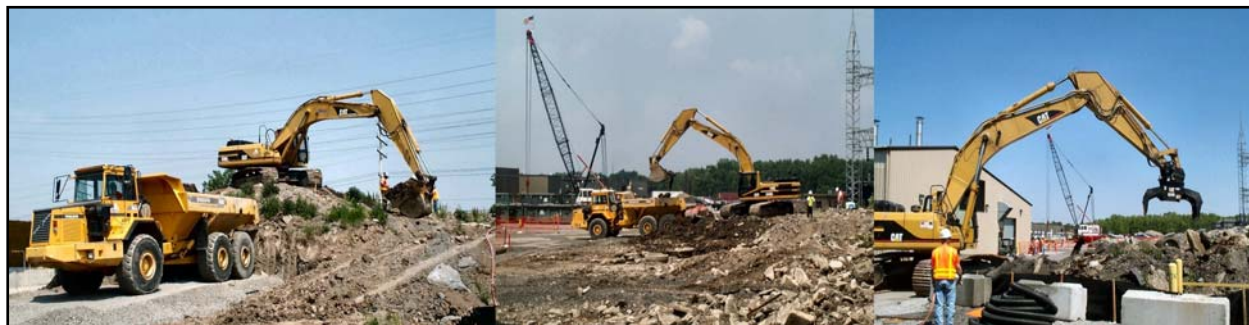
Figure 2 – Conventional excavation techniques were used to relocate spoils pile materials.
