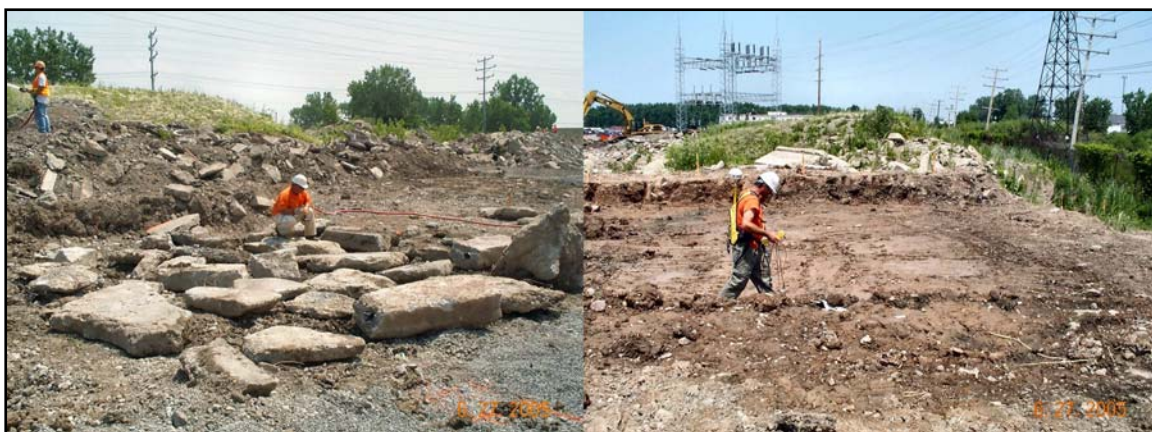
Figure 3 – Health Physics Technicians performed daily scanning of spoils pile material.
