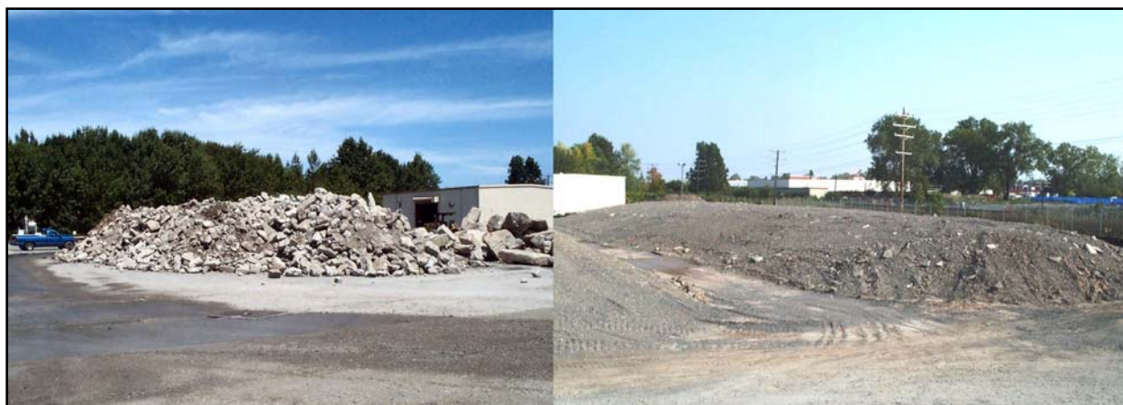
Figure 4 – Relocated materials were separated according to composition (concrete, soil, debris) and were placed in designated staging areas prior to removal off-site.
