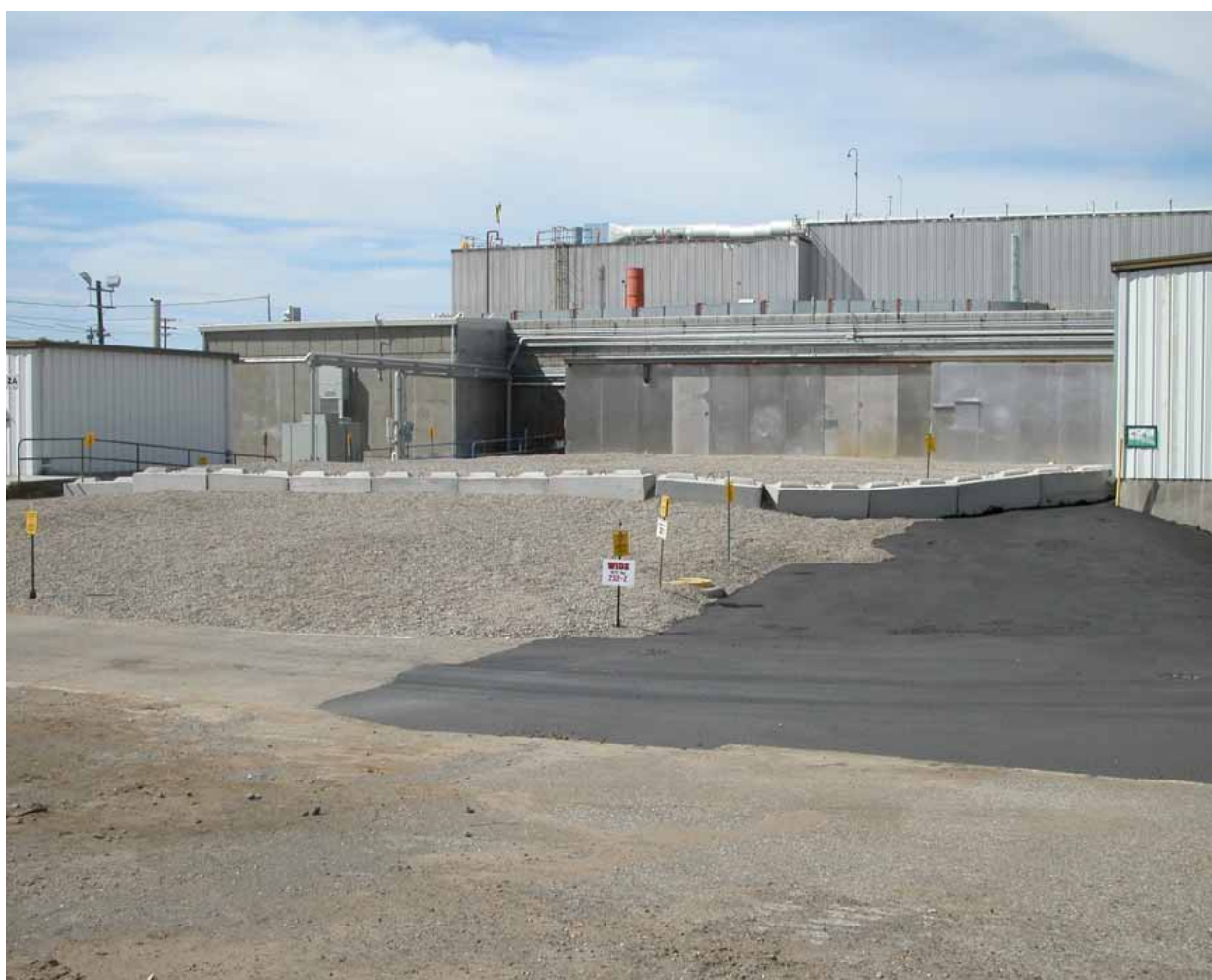
Fig. 4. When the project was completed the facility had been removed and a cap installed to prevent contamination from migrating to the environment.
