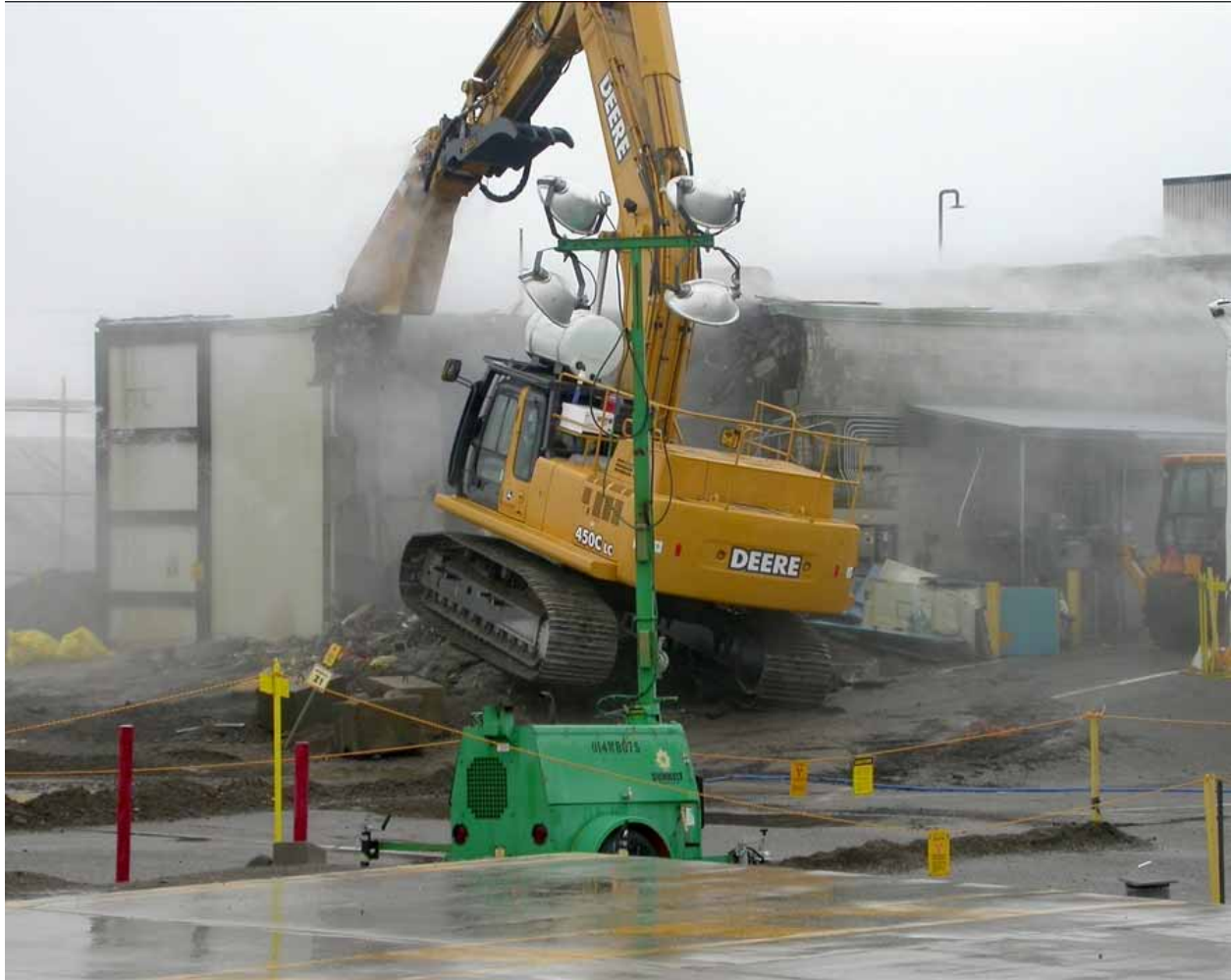
Fig. 3 Misting equipment was installed on 232-Z, the surrounding buildings, and the demolition excavator.
