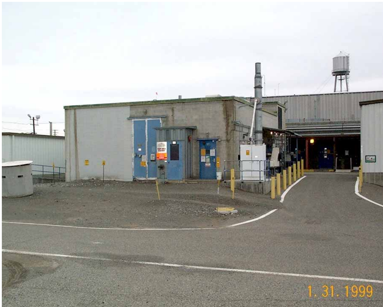
Fig. 1. This photo shows the 232-Z Facility and nearby buildings before demolition.
