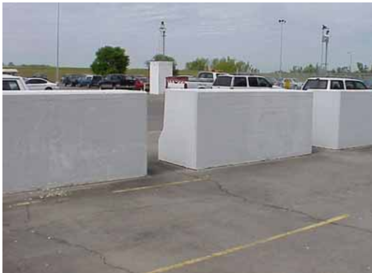
Figure 3 – High energy capacity/high deterrent, surface mounted precast concrete inertia vehicle barrier system
