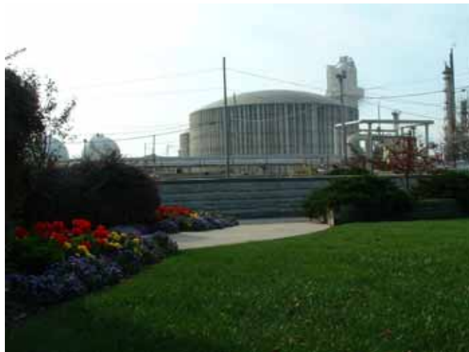
Figure 1 – Cast-in-place reinforced concrete wall designed to appear as masonry, serving as a high energy capacity vehicle barrier
