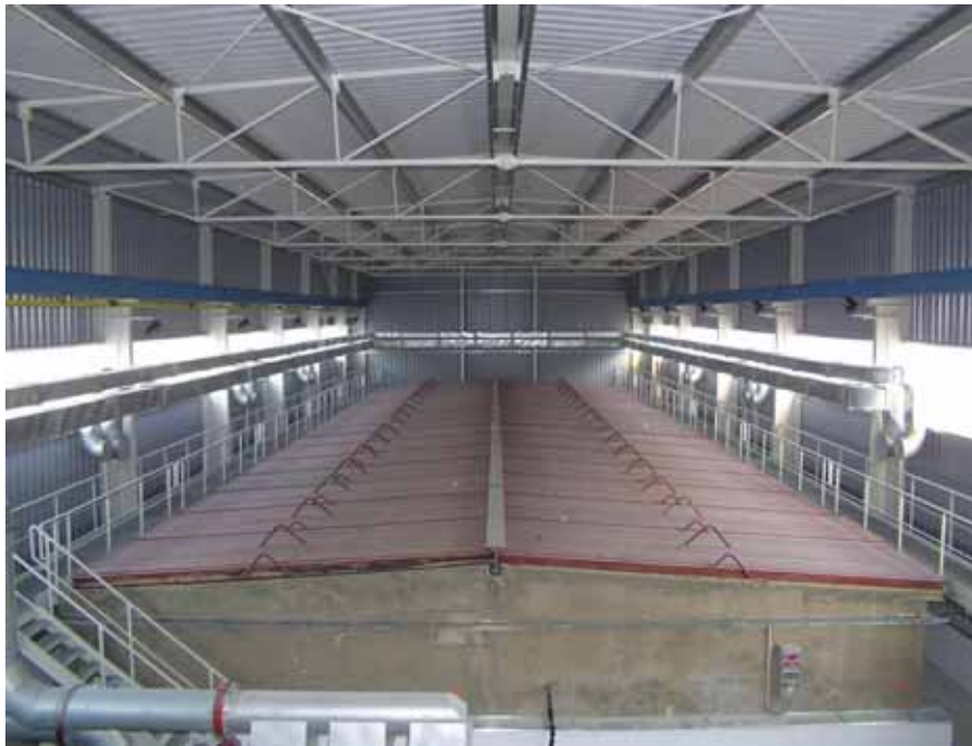
Fig. 3. Building No. 211/6 – Reloading Site with a new hall
