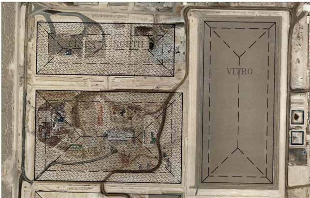
Figure 1 Aerial view of EnergySolutions Clive site with Class A, Class A North
