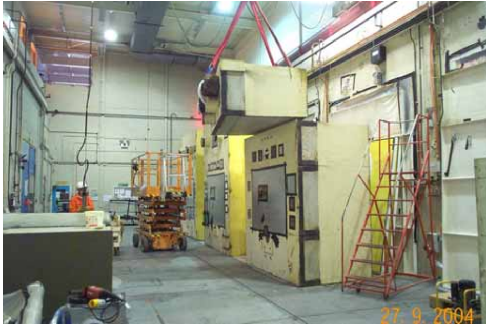
Figure 1: Removal & dismantling of cave line modular shielding blocks with the north cave line on the right and south cave line on the left looking west surface swabs and counting them in a low background position. The end point was reached after a series of decontamination sweeps over all internal surfaces showed that no further reduction in mean dose rate could be achieved.
