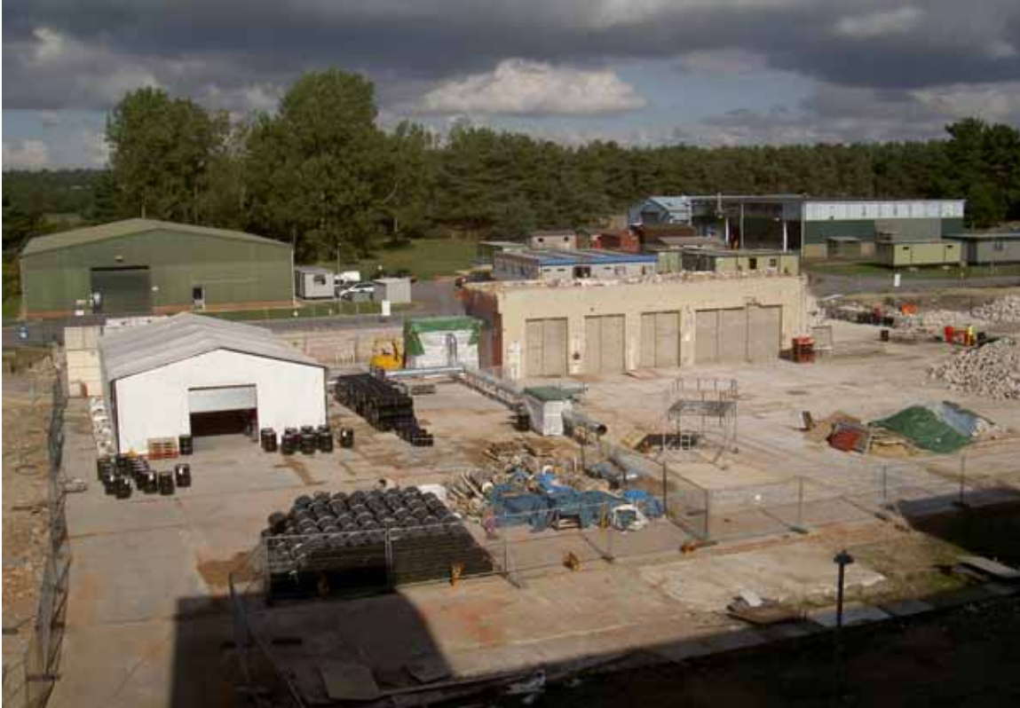
Figure 4: Demolition site showing HAKI tent and remains of north cave line plus the ventilation system and horizontal discharge stack
