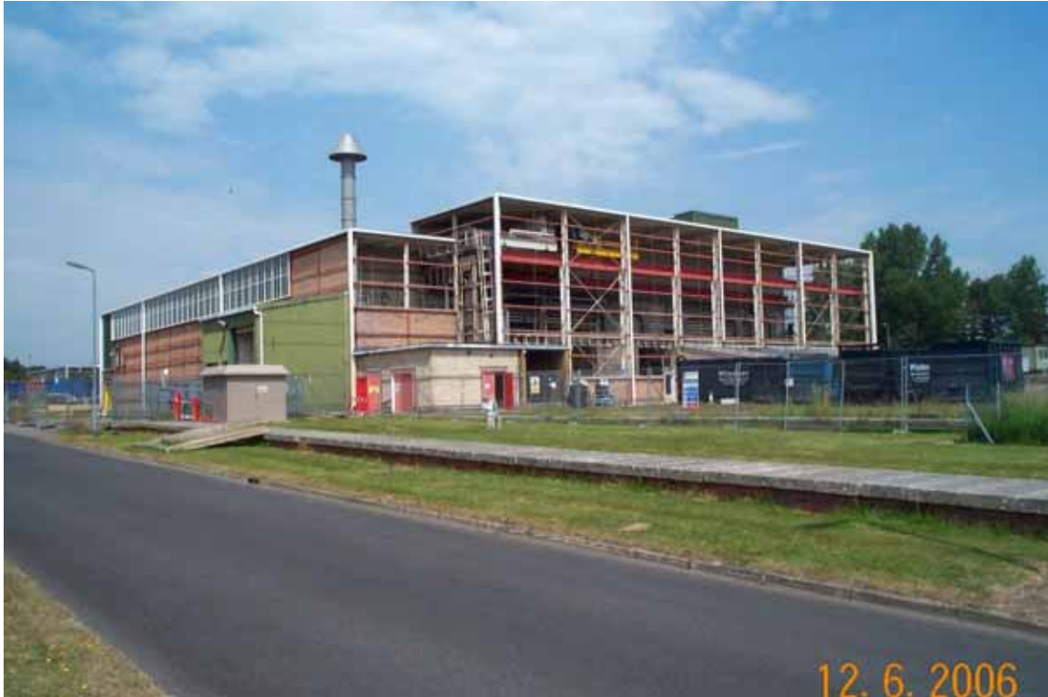
Figure 3: View of the building after removal of the concrete asbestos cladding
