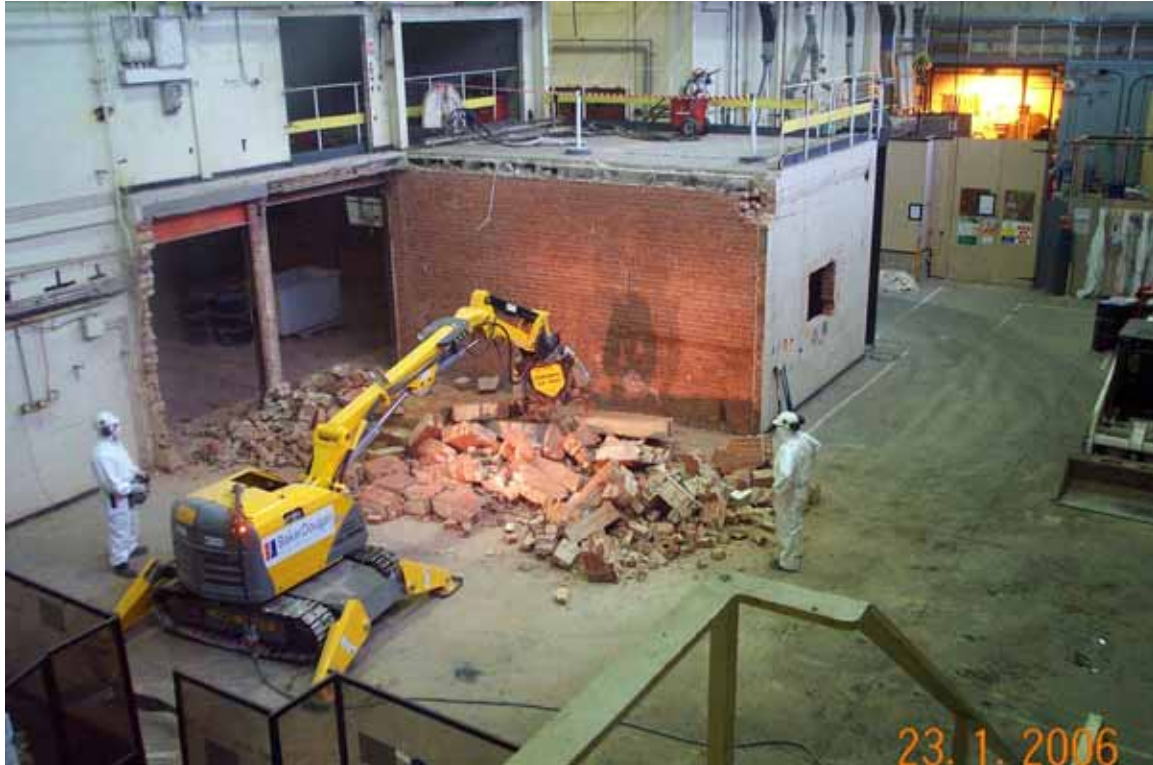
Figure 2: Demolition of pressurised suit facility using BROKK 330 unit
