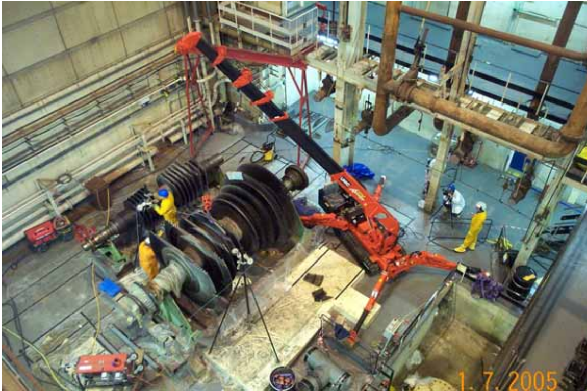
Figure 1: Diamond wire-sawing LP rotors for loading into ISO container for disposal
