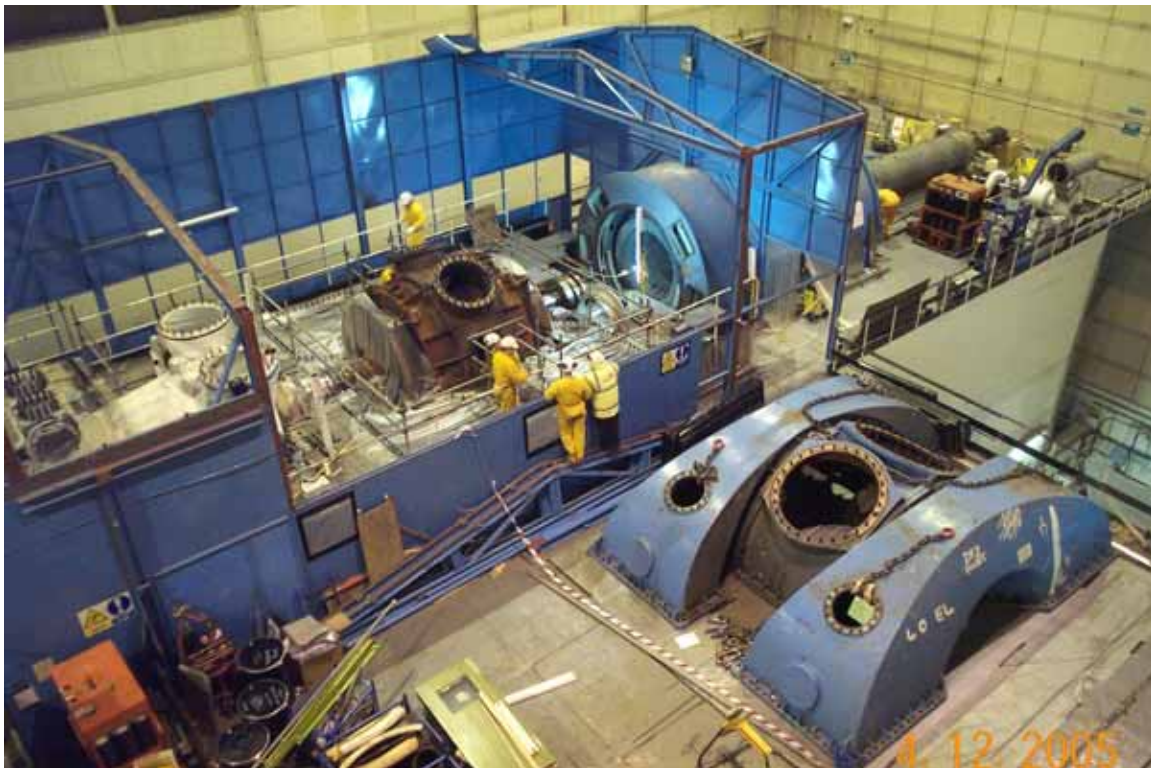
Figure 2: Dismantling the steam turbine and alternator sections of the generator
