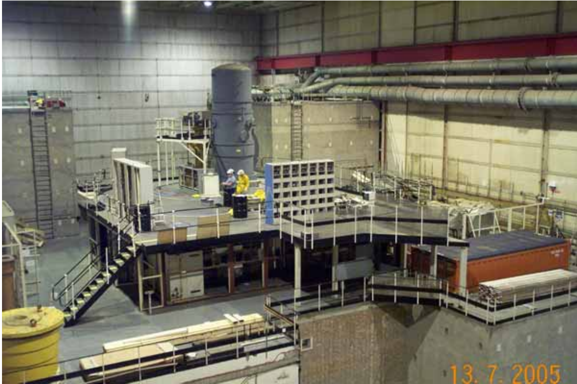
Figure 3: Early stage view across Turbine Hall to Refuelling Machine
