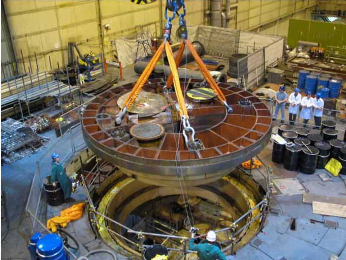
Figure 4: Lifting out the inner section of the Rotating Shields
